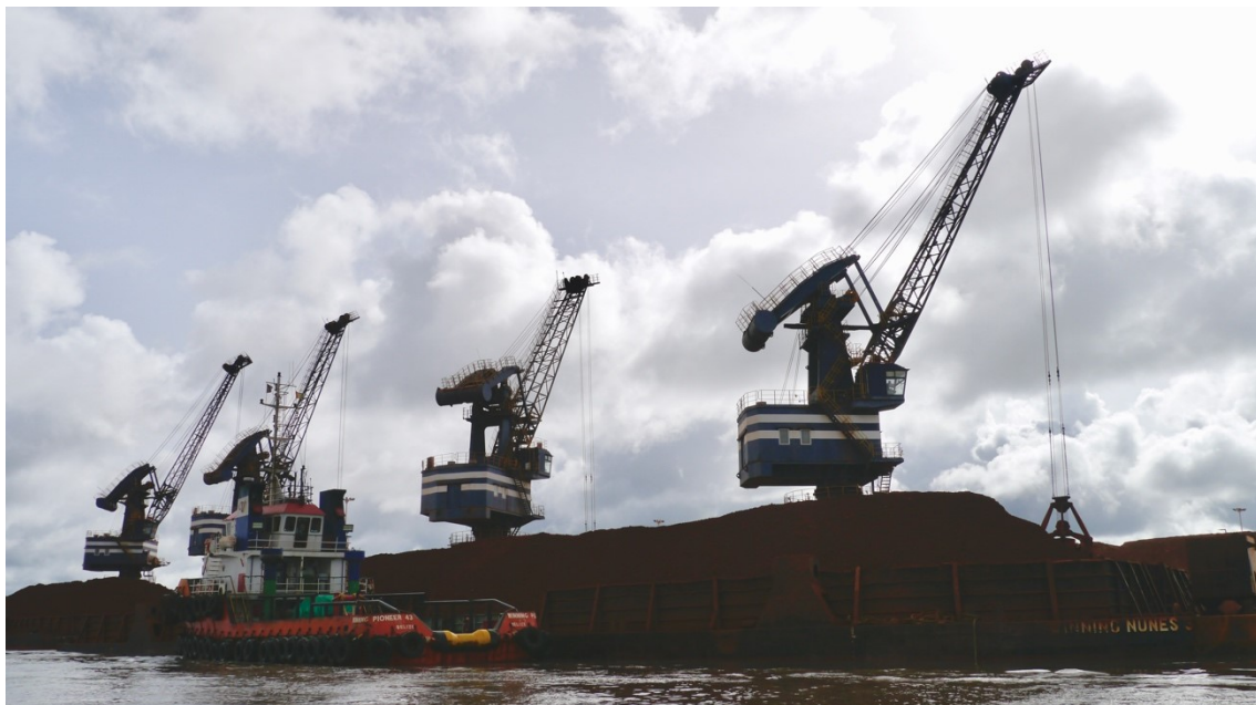
Figure 3. Barge Loading Facilities in Guinea.
